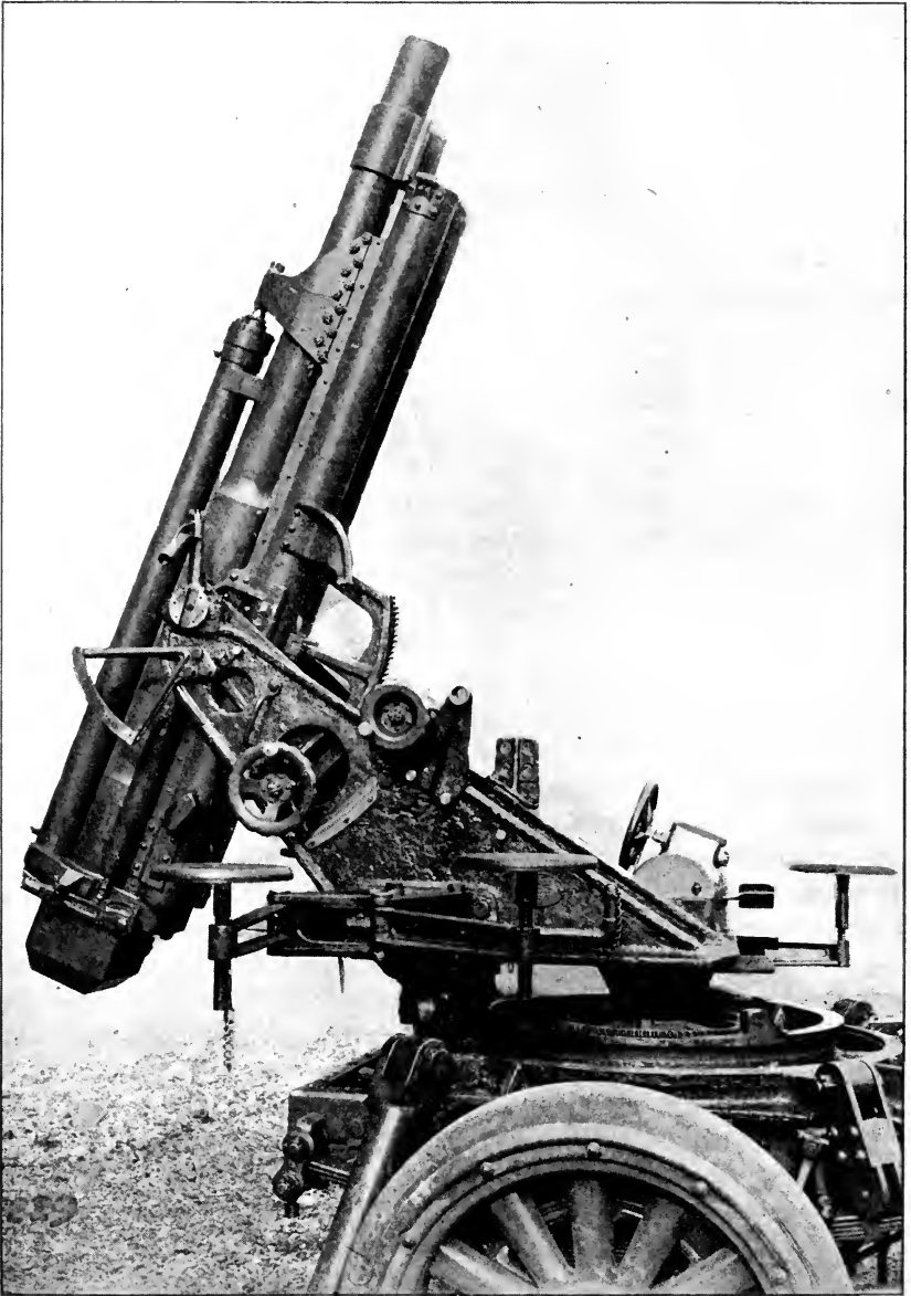
GUN MOUNT SHOWING GUN AT MAXIMUM ELEVATION.
